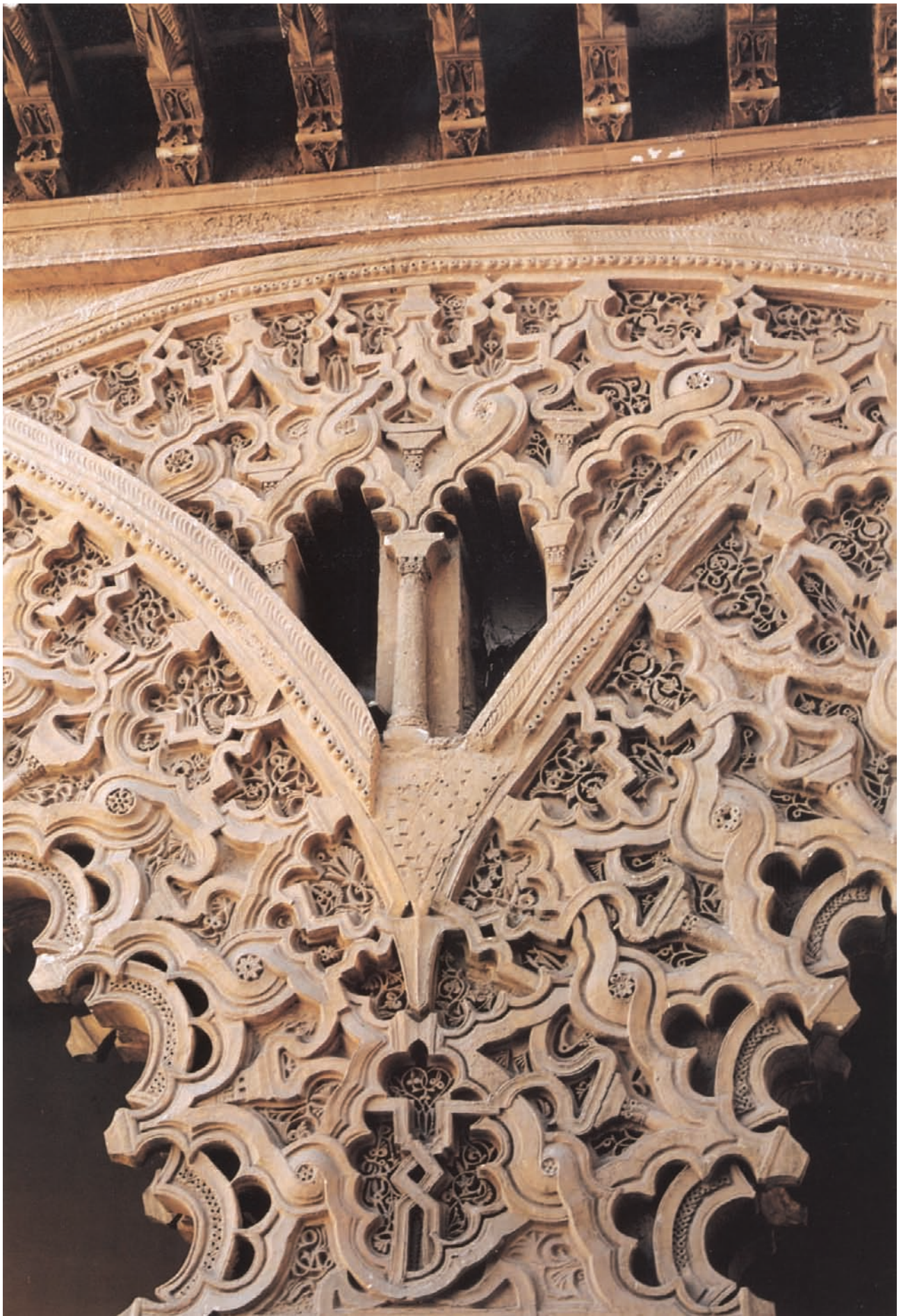
Fig. 10 Saragossa, Aljafería, intersecting arches in courtyard, detail
