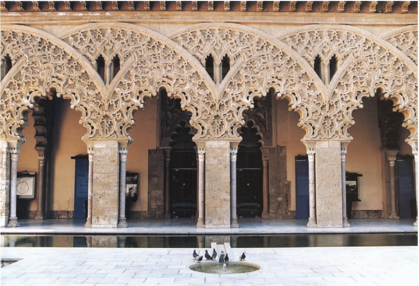
Fig. 9 Saragossa, Aljafería, intersecting arches in courtyard
